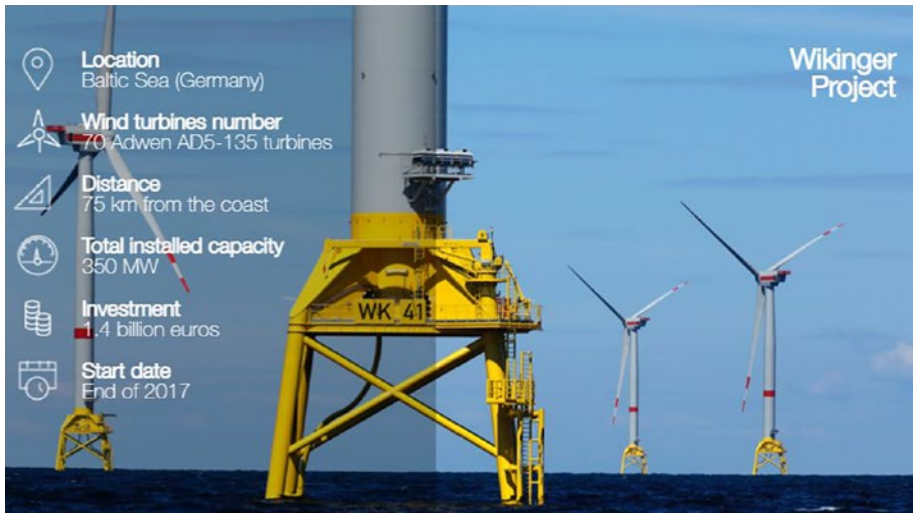
Figure 12-1. Wikinger offshore wind farm. Source: iberdrola.com [14]
