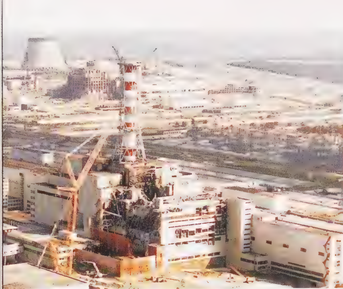
Figure 16 An explosion occurred at the Chernobyl reactor in the Ukraine after graphite control rods caught fire. The explosion shattered the reactor's roof.
