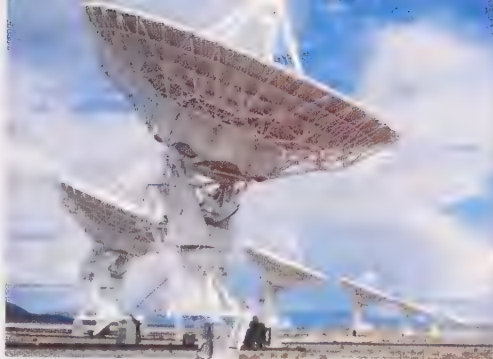
Figure 4 27 dish antennae of the VLA are mounted on railroad tracks for rapid repositioning. The 304-m dish antenna in Arecibo, Puerto Rico is shown in the inset.
