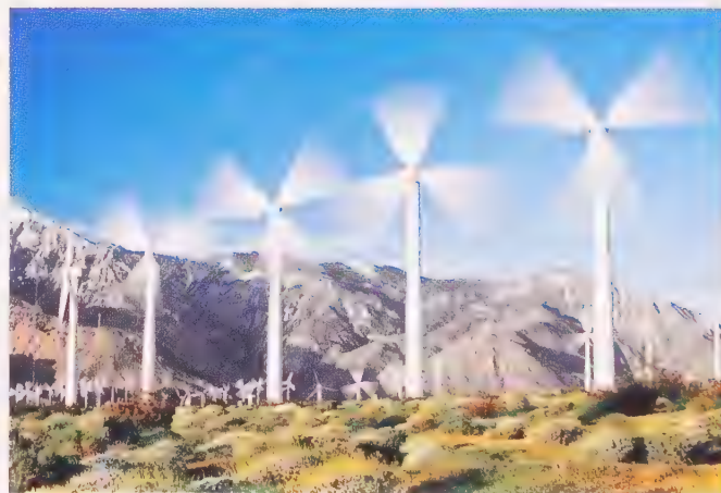
Figure 19 The propeller on each of these windmills is connected to an electric generator. The rotating propeller rotates a coil or a permanent magnet.
