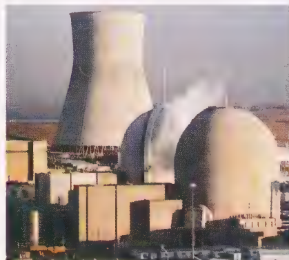
Figure 11 A nuclear power plant generates electricity using the energy released in nuclear fission. Each of the domes contain a nuclear reactor. A cooling tower is on the left.
