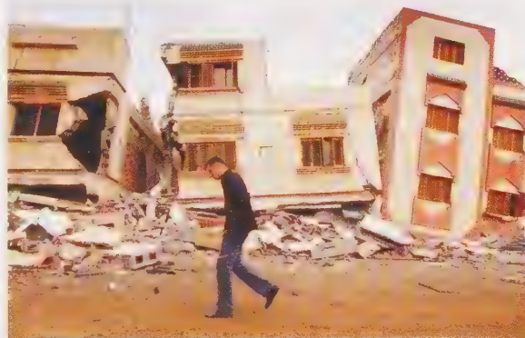
Figure 13 This damage was caused when the buildings were shaken off their foundations.
