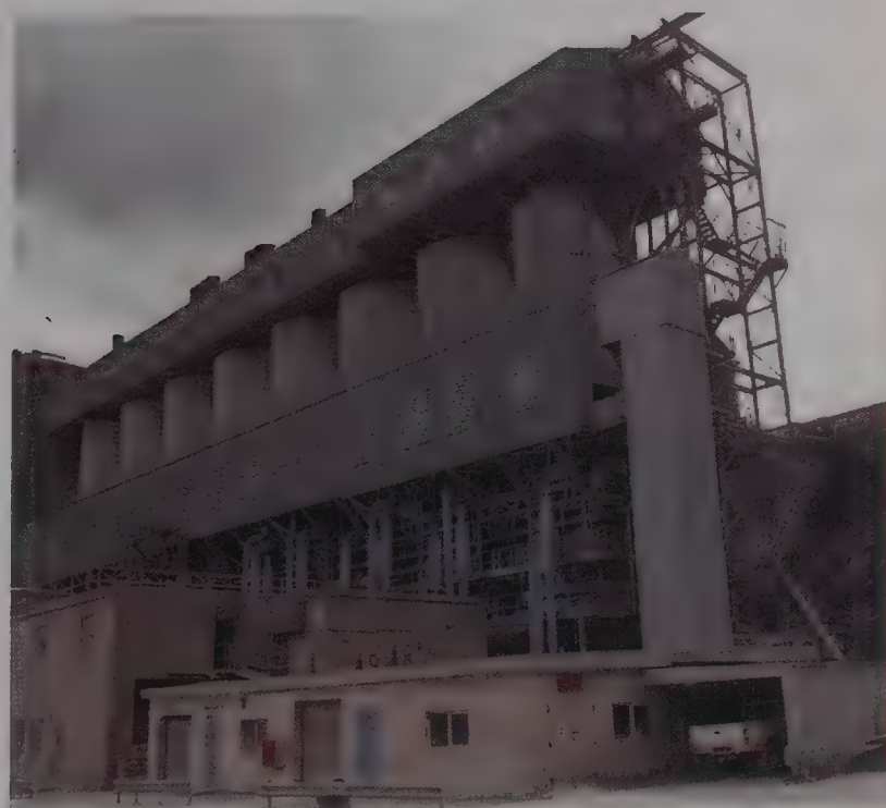
● Figure 13.2 A modern lime kiln. Calcium carbonate, as limestone or chalk, has been converted to calcium oxide (quicklime) for centuries (see page 71), by strong heating in lime-kilns.
